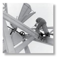
blades and they do not turn. When the wind changes direction it will blow more sideways-on to the fantail and will cause it to turn. The fantail, driving through a gear mechanism inside the cap, causes the cap of the mill to turn until the sails are facing into the wind again.
