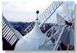
As the cap frame merely rests upon the curb there is a tendency for it to slip sideways off the tower when the fantail drives it around. To prevent this there are 12 centring wheels, each about 30cms in diameter, fixed to the underside of the cap frame and locating just inside the curb.
