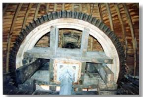
tower down to the gallery. When the miller raises the lever the brake band is slackened off and the sails may turn. When he lowers it, the band tightens around the brake wheel, bringing the mill to a stop.
